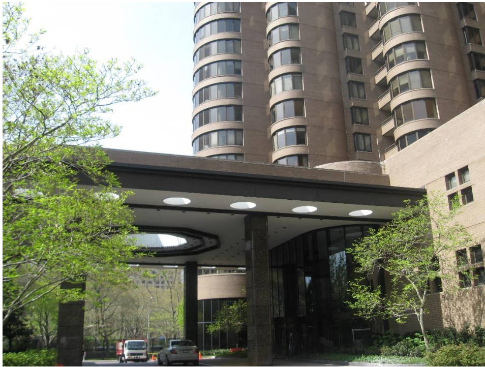
The Corinthian building entrance (own photo)
