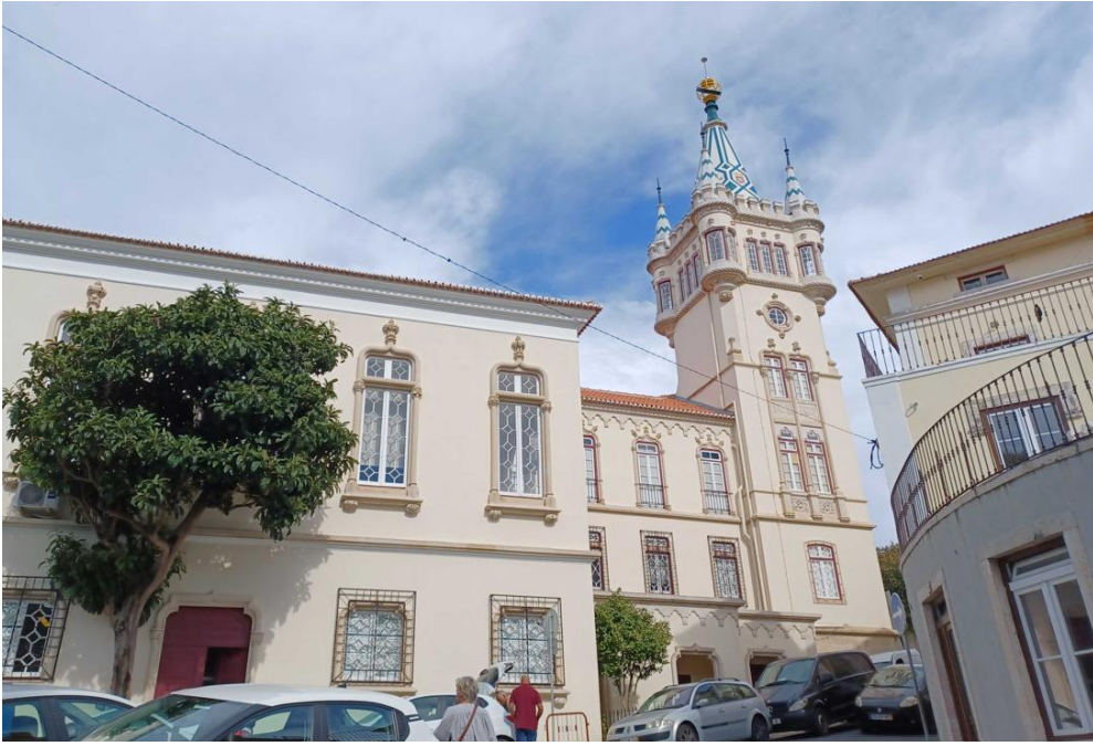
The side of the town hall
