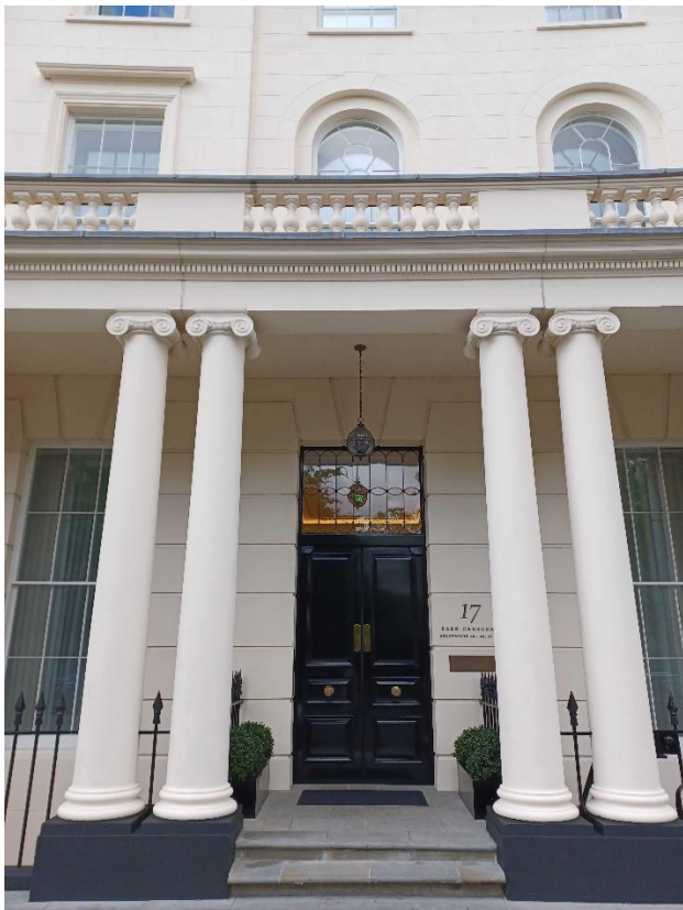
Detail of an entrance door
