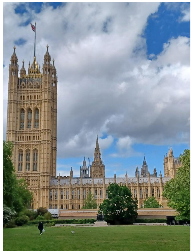
Back of Westminster Palace, as seen from Victoria Tower Gardens
