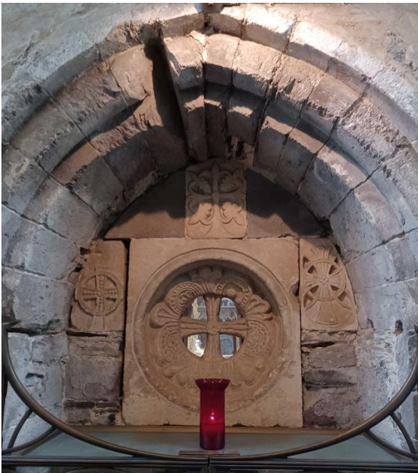
The cross niche in the old exterior wall on the 12 th -century cathedral
