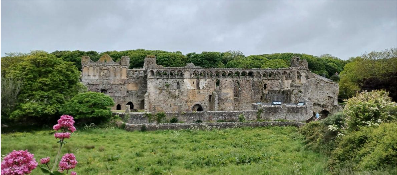
General view of the Palace
