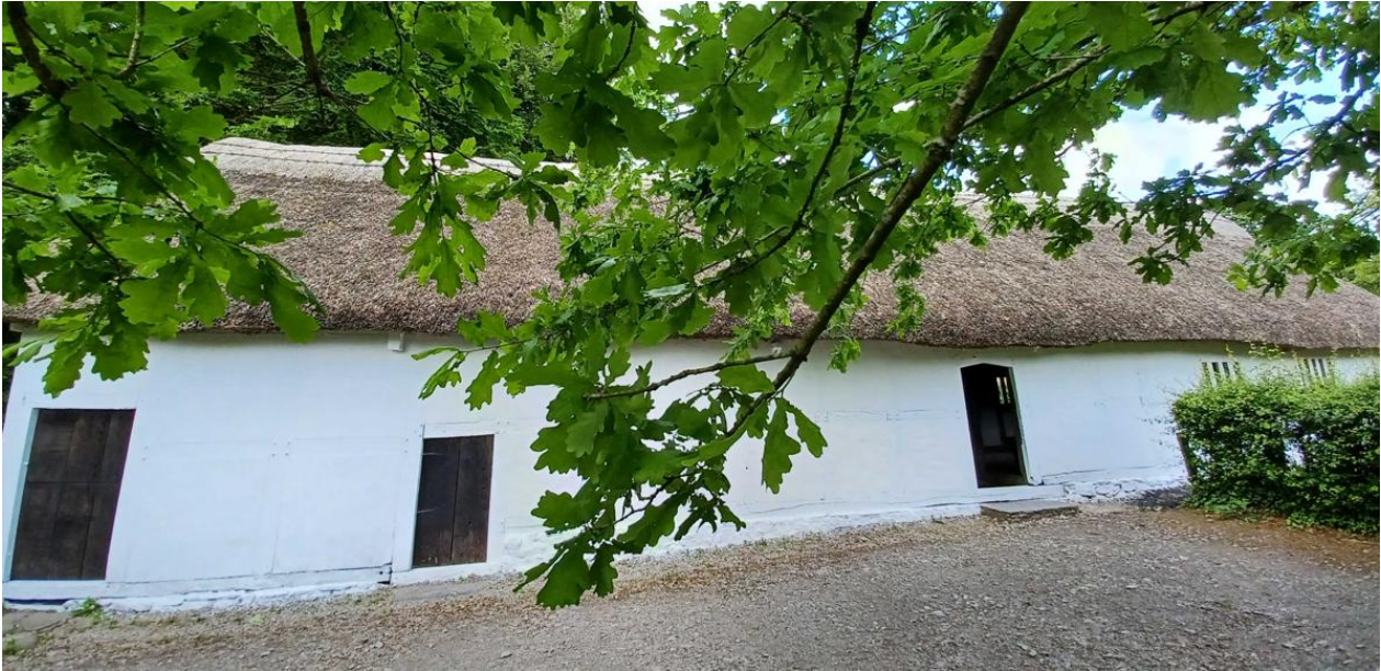
The front entrance of the house
